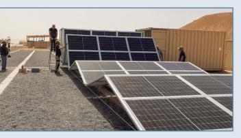
Currently installed on a Middle East Air Base as part of Operation Chammal, the KAPI solar/battery/diesel hybrid power plant effectively reduces the base's fossil energy needs.
